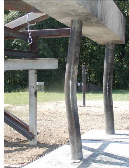
Figure 3. Bent 1-C5 (#5) after the test.
